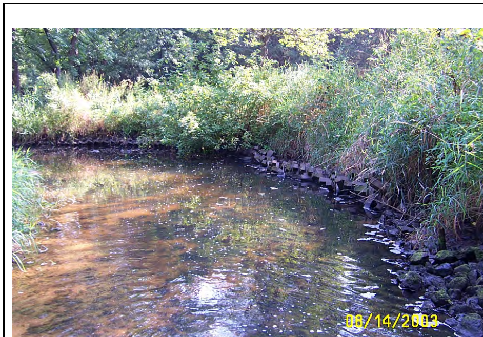
Figure 5-31 Reach PC7B Bank Stabilization Site
